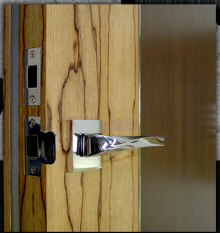
Double Contemporary Flush Door with Qtrs. African Mahogany and White Ebony Veneers, Vertical Bookmatch Valli and Valli Hardware, Fusital Collection, Privacy Set with bolt. Polished Chrome (US26). White Ebony Veneer Astragal 13.2
